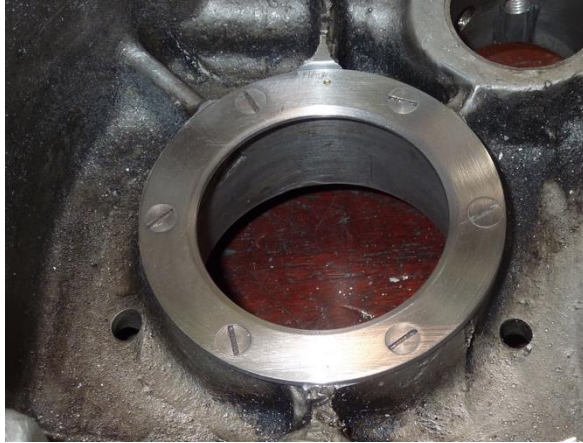
Replacement ring in position
